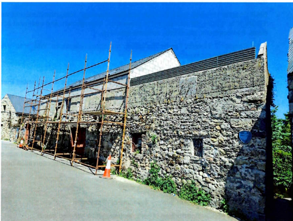
Figure 2-3. Current state of building previously marked PR2 as of 25/05/2026
