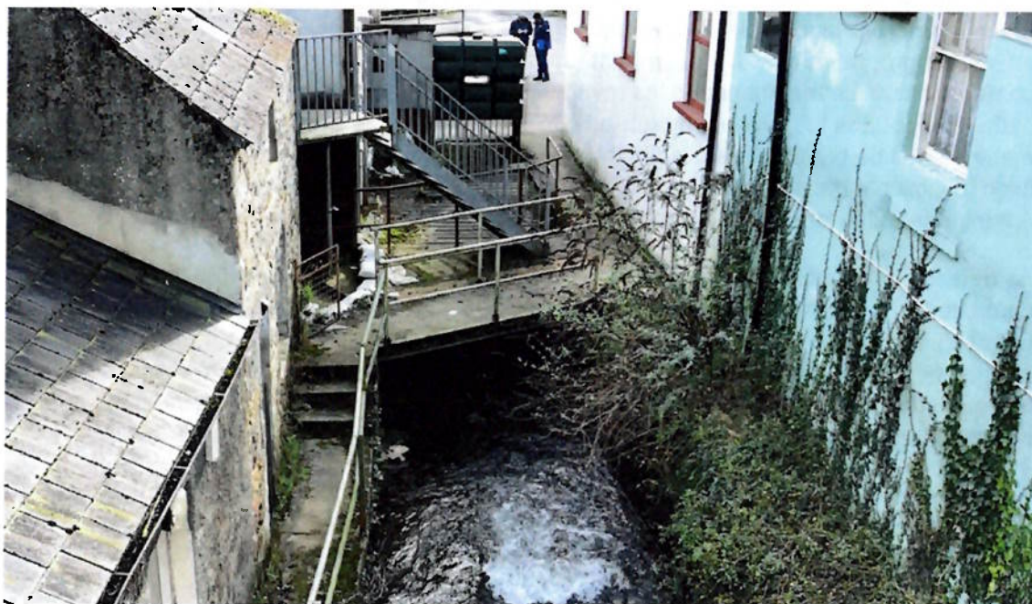
Figure 2-4. Bridge (in the foreground) to be replaced at Turf Market
